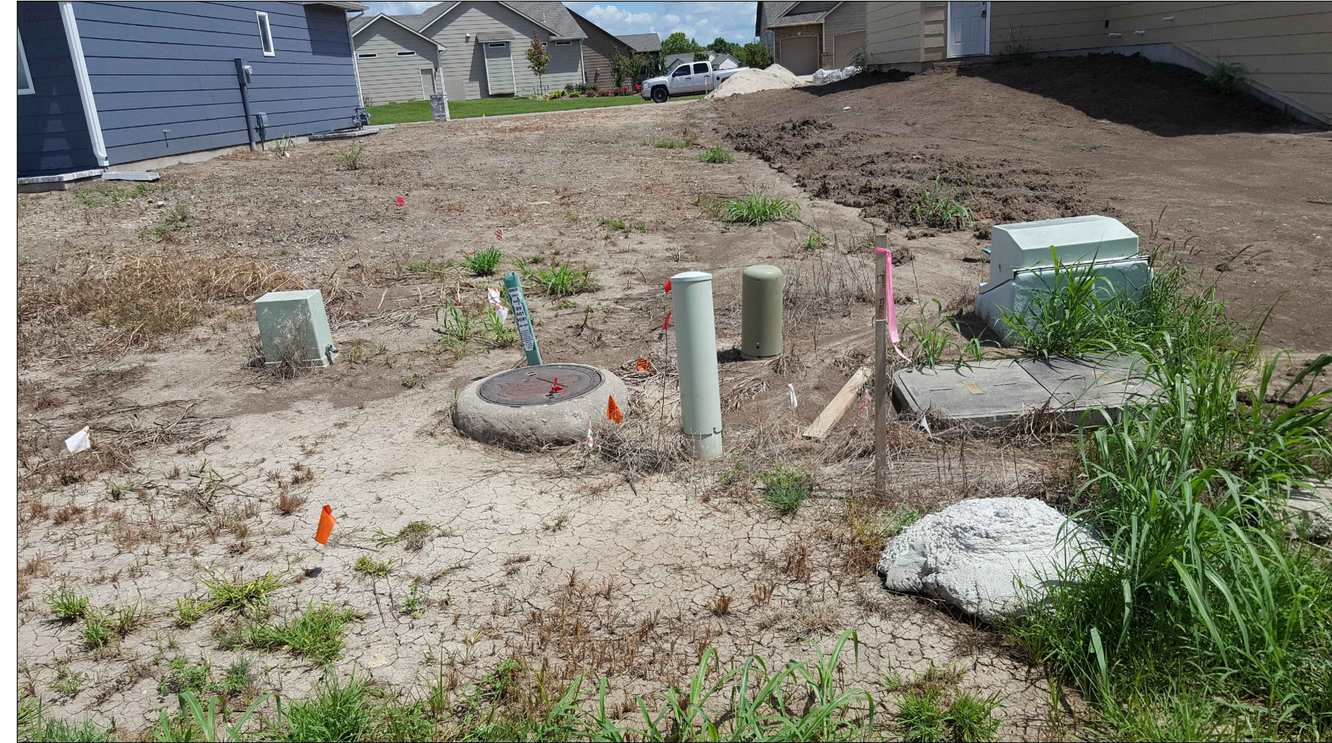
Figure 2 Photograph of Existing Manhole in Lot 22, Block 4 from the southwest viewing toward the northeast. Note the nearby utility structures and concrete waste. See Sheet 8.
