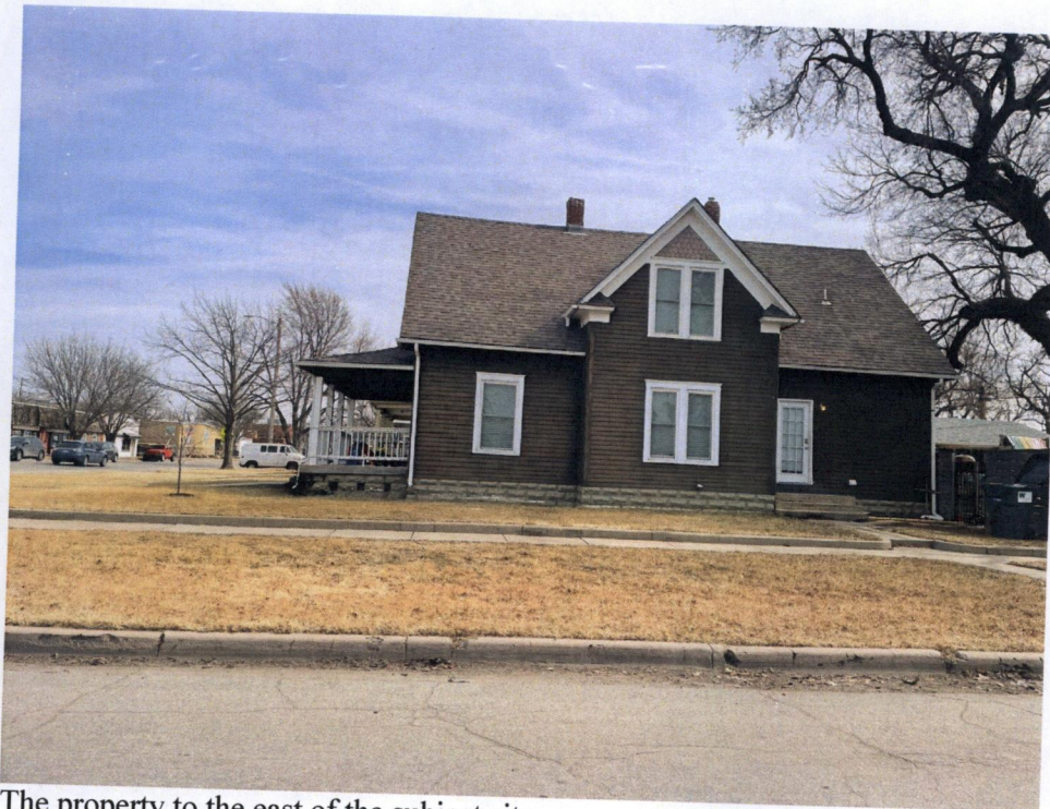
The property to the north of the subject site
