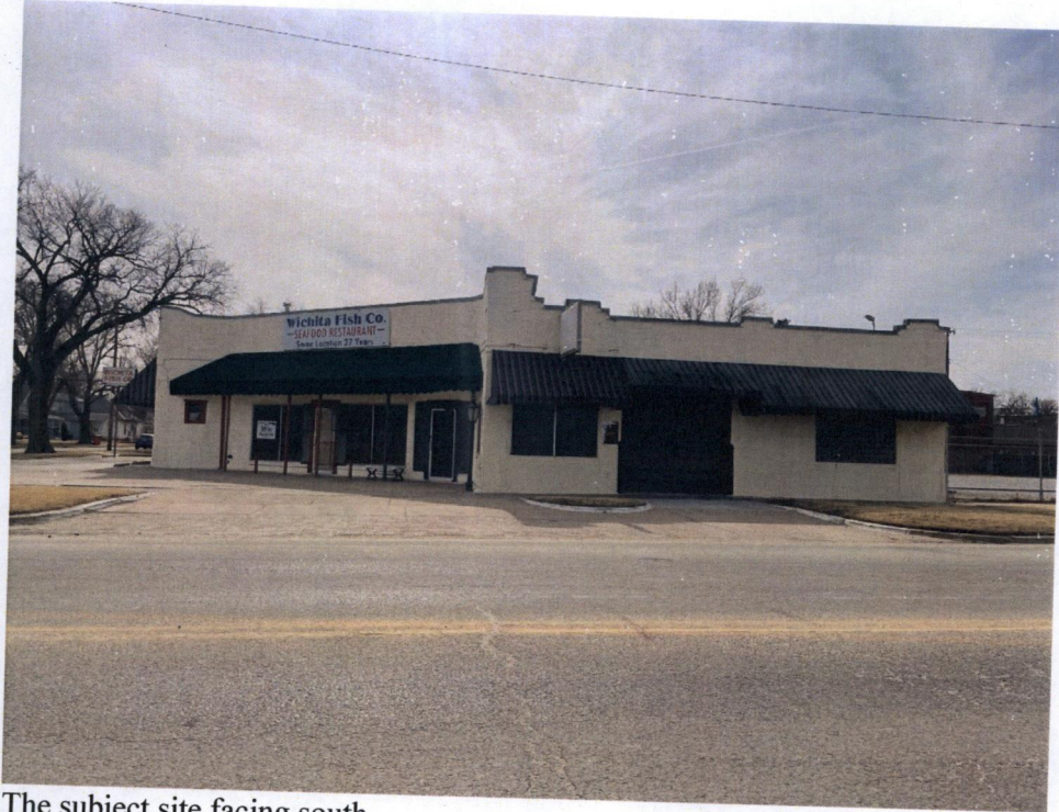
The subject site facing south
