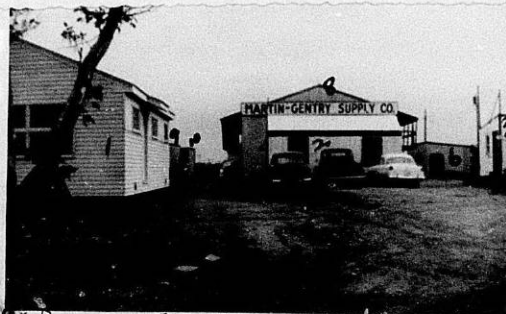
4x D Front View from 31st St.
