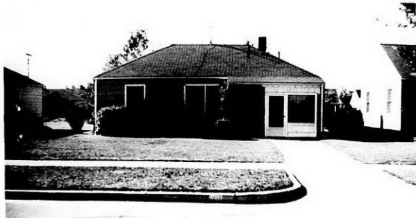
Exterior view of remodeled garage at 1927 Swan Street
