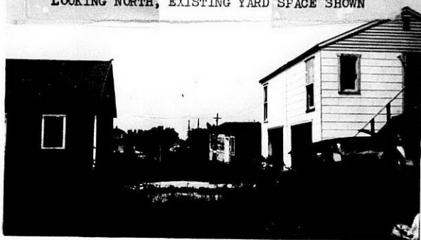
LOOKING NORTH, EXISTING YARD SPACE SHOWN
