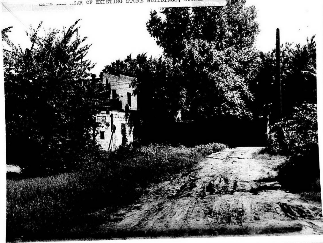
BACK AND REAR OF EXISTING STORE BUILDINGS, LOOKING SOUTH
