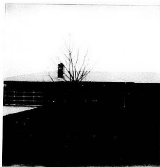
WESTERN QUARTER 1100 FEET, ONE HALF MILE NORTH, DIRECTLY EAST OF THE PROPOSED 11-DEGREE ROAD ON EAST GENERAL AVE.
