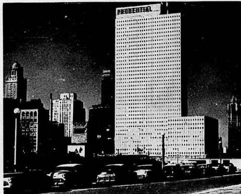
PRUDENTIAL REGIONAL OFFICE BUILDING — CHICAGO, ILLINOIS (Survey 1951) Building Completed 1955
