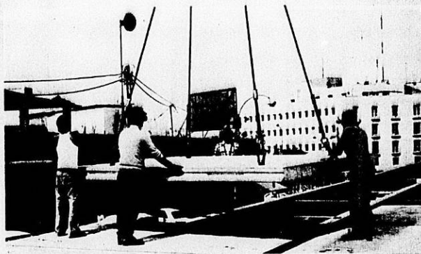
(3) Concrete slabs weighing 2.7 tons (2.5 m) are fastened tightly to the metal structure. Slabs are standardized and identical.
