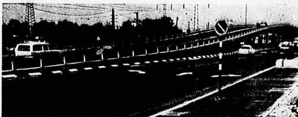
(1) AB Bridge 1 (named for its designer) in Brussels, Belgium was inaugurated in February 1975. It provides three traffic lanes over a busy intersection. The main span over the intersection is 117 ft (35.7 m); overall length is 1411 ft (430 m). The metal superstructure was secured in four hours.
