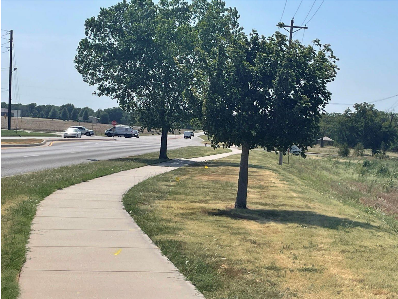
Sidewalk and power poles in the West 29 th Street North right-of-way abutting subject site (facing southwest)
