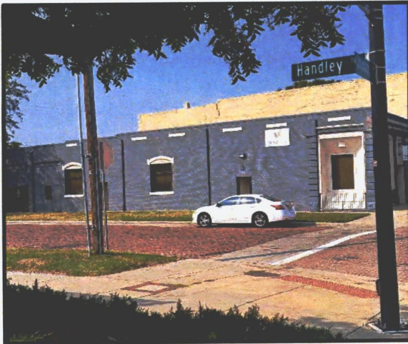
East side of building at 901 W. Douglas
