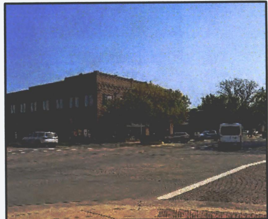
Northeast corner of Handley & Douglas -BBQ shop
