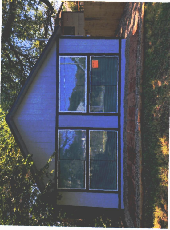
Looking east towards accessory structure
