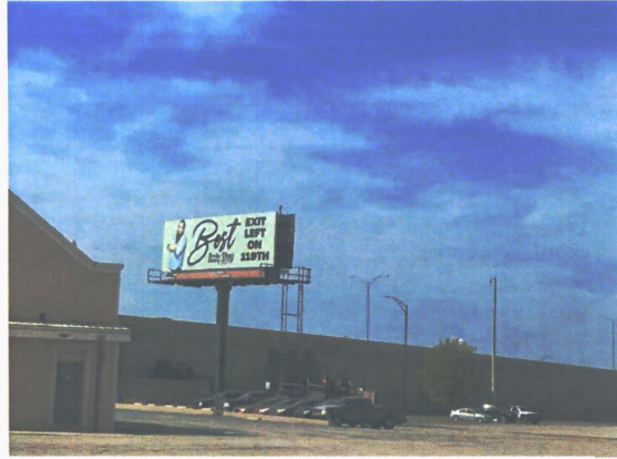
The subject sign and site.
