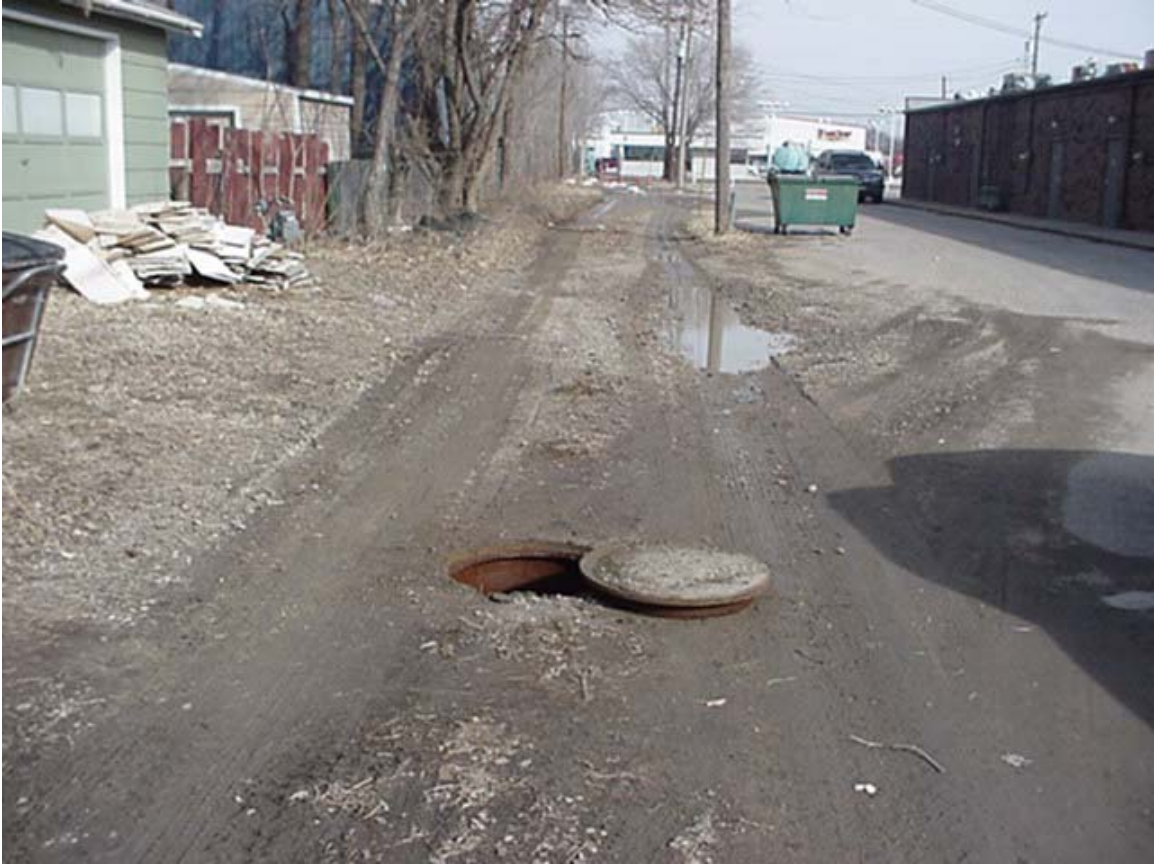
Standing south of MH 5547-404, looking north.
