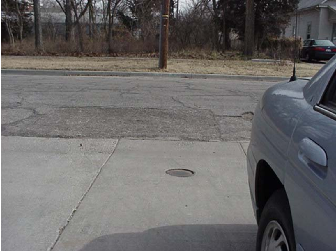
Standing west of Glenn Street R/W, looking east.
