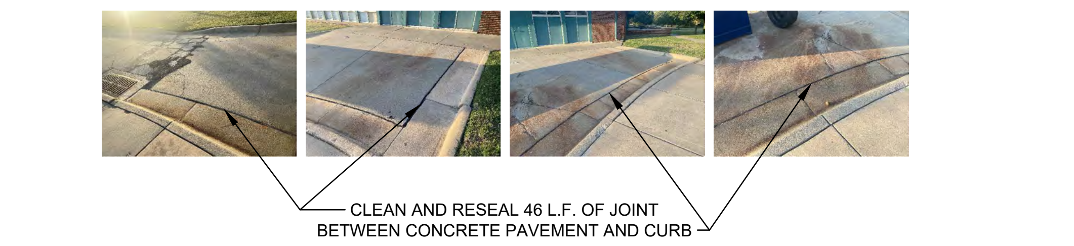
H SERVICE DRIVE REPAIR SCALE: NONE
